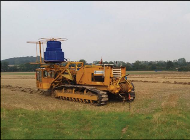
and we raised the depth of the new drains to prevent damaging the existing ones, whilst old drains were not working well there is little point in damaging something which is moving some water.
